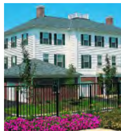
The balcony railing shown on roof top is Series 990 with Superior panel column posts. The railing shown in foreground is Series 900.
